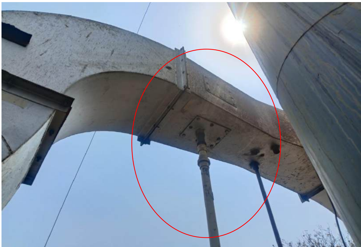
Water pipe with pores provided inside the vent connecting Hot Mix Plant and stack for scrubbing.
